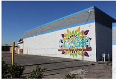
BUILDING WRAP MADE UP OF VERTICAL PANELS-(SPANELS)
